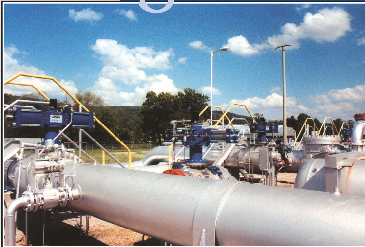
The Gevalco "Remote Electric Control" module is designed to meet the need to operate pipeline valves from a remote electric signal.
