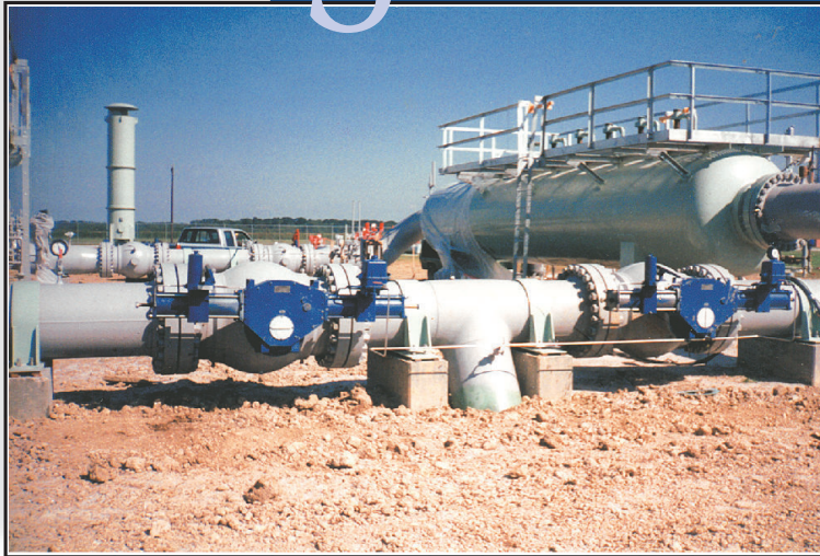
With working pressures up to 3000 psig, the Gevalco "Dual 3-way Poppet Control Valve" utilizes the direct pipeline pressure gas for both power gas and pilot media...
