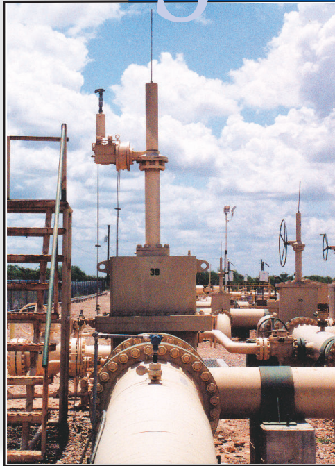
The Gevalco "Gas Motor Actuator Control" package utilizes hi-pressure poppet valve technology to provide reliable, maintenance-free control of gas motor actuators.
